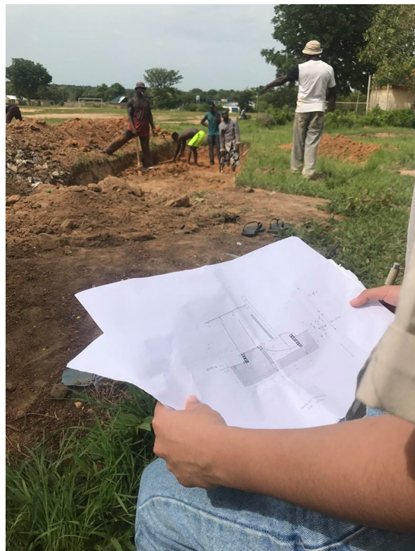
Figure 5.1: The toilet construction site
