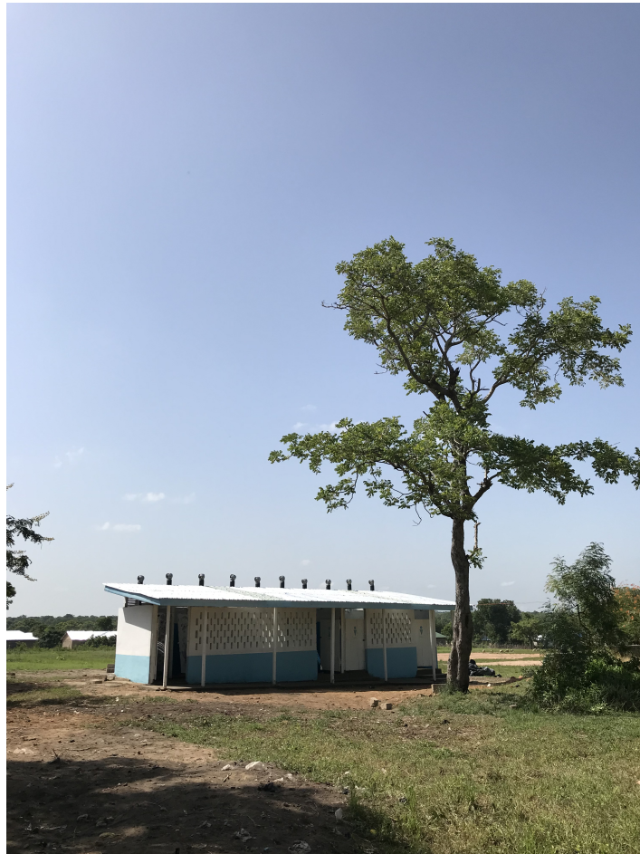
Figure 19.1: The completed toilet
